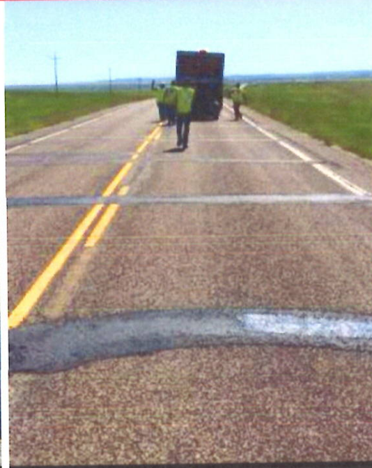
Leveling Depressed Thermal Cracks
