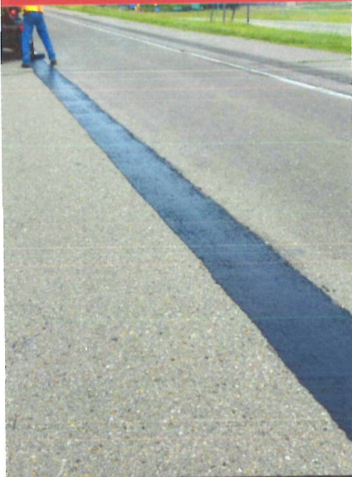
Repairing Deteriorated Longitudinal Joints
