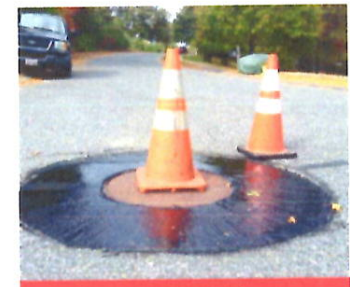
LEVELING MANHOLE COVERS
