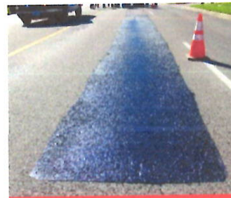
SKIN PATCH REPAIRS
