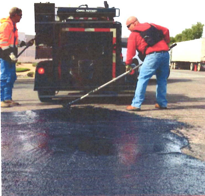
PRETREATMENT OF FATIGUE CRACKED AREAS PRIOR TO SURFACE TREATMENTS
